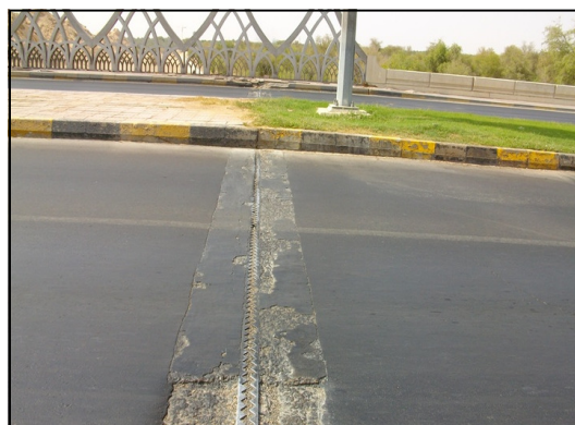
Failed joint
