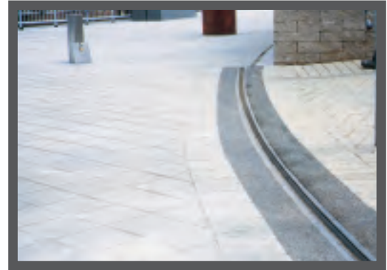
The Advanced EMR bridge joint system installed to radius.
