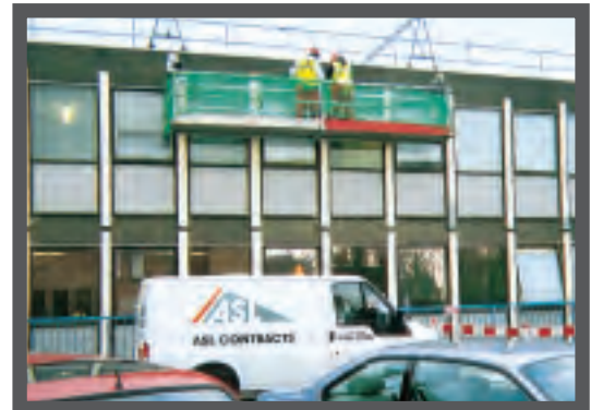
Undertaking concrete repair and anti carbonation works.
