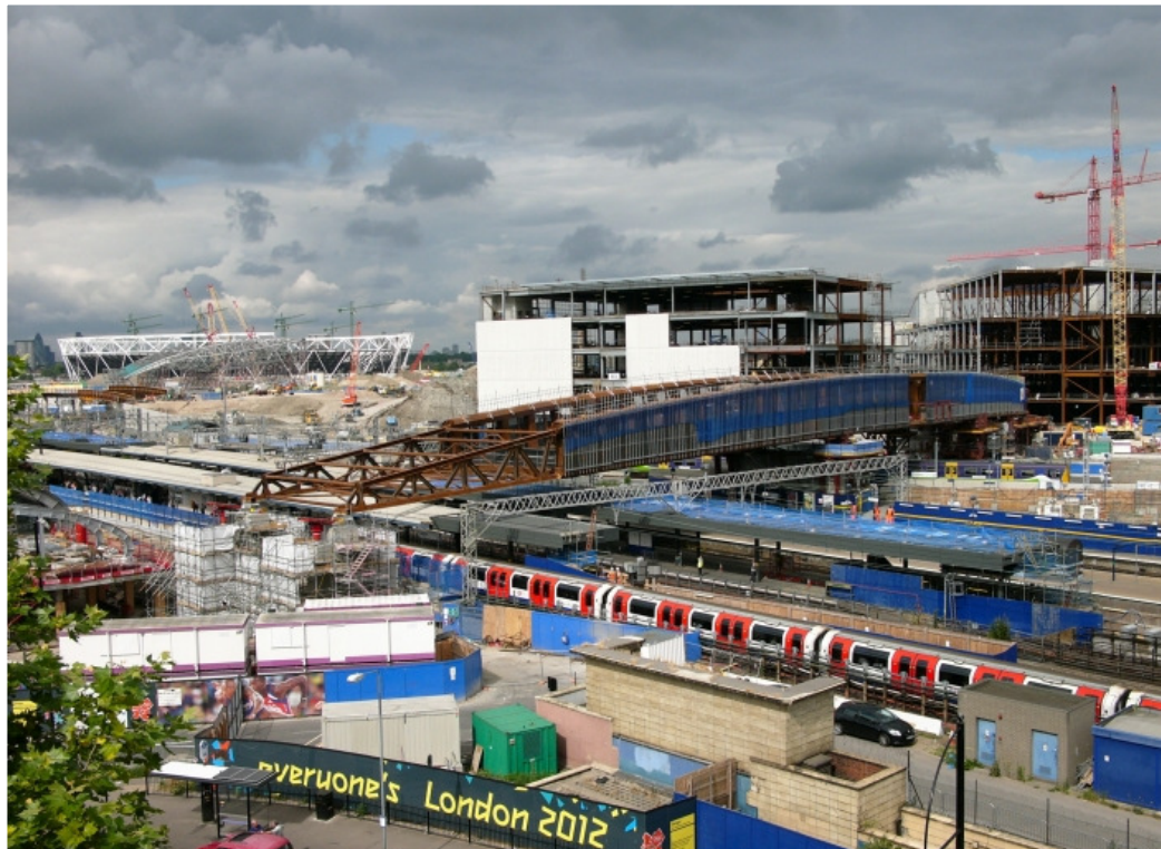
Bridge 17 Over Woolwich Line April 2010
