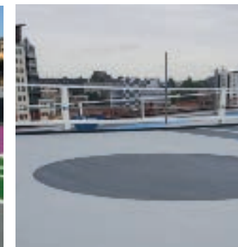
Ramps & Turning Circles
